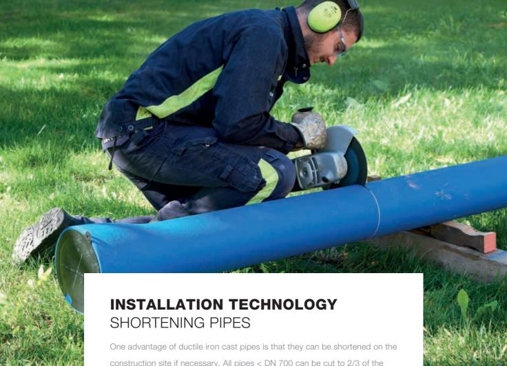
construction site if necessary. All pipes < DN 700 can be cut to 2/3 of the construction length, measured from the insertion end, and have no marking. Cut pipes >DN 700 are supplied on special order. The weld bead required for the restrained socket joint has to be reapplied using the electrode specified by the supplier.
